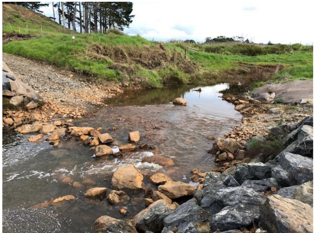
5 th June, 2020, Dam and rock walls still in place Photo: Jenny Price
