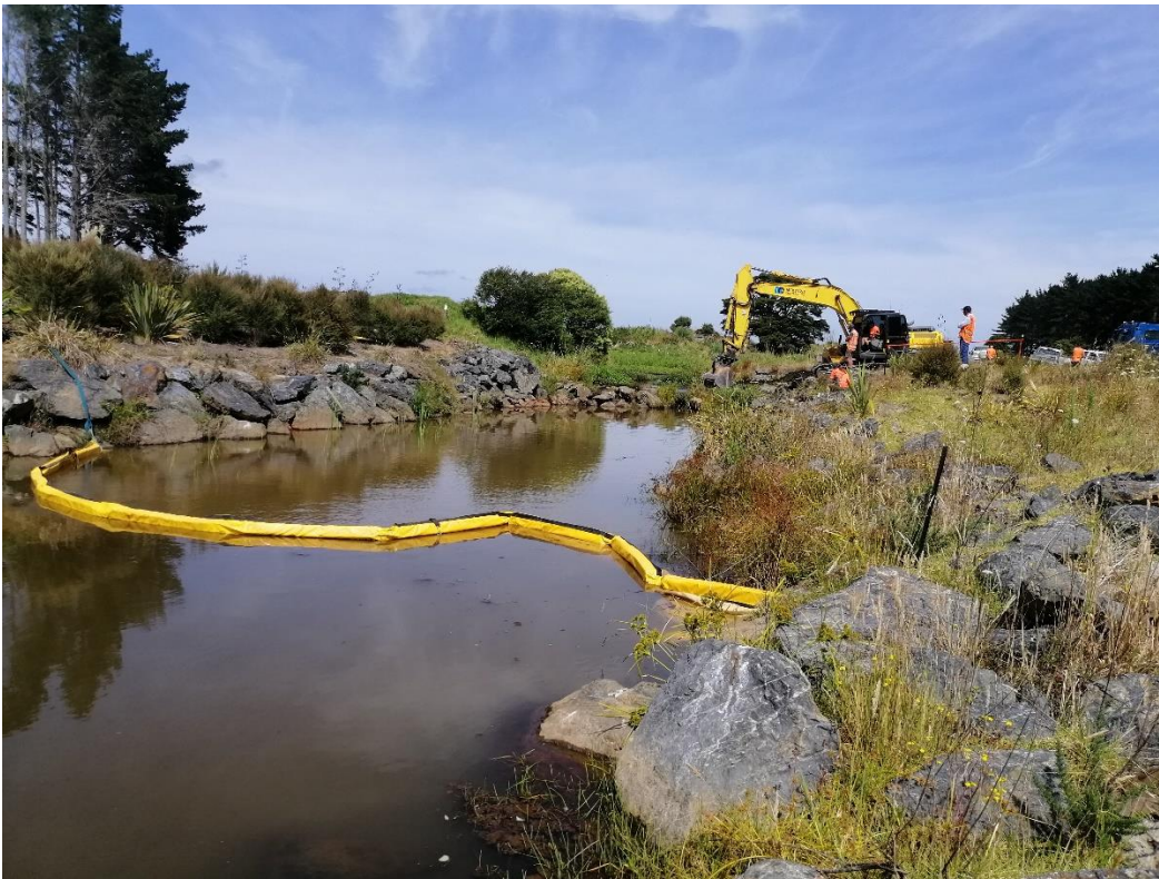
The boom downstream to trap sediment
